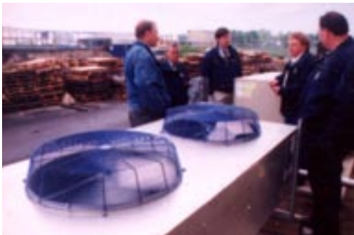
Larkin units provide tight temperature control to ensure product quality. (Pictured left to right): Paul Clement, of Controlled Environmental Systems, Jim LaPierre of Refrigeration Sales Inc., Tod Heath of Miller Component Sales, Dean Betlee of Controlled Environmental Systems and Jon Dresser of Refrigeration Sales Inc.
