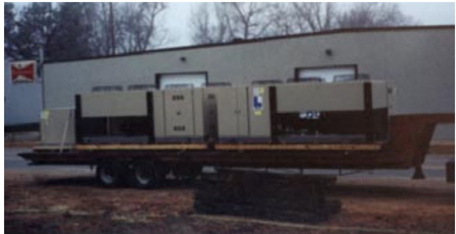
James Sims, with R&E Supply, recommended that Larkin units be installed at the M&K Distributors center in Pine Bluff, Arkansas.
